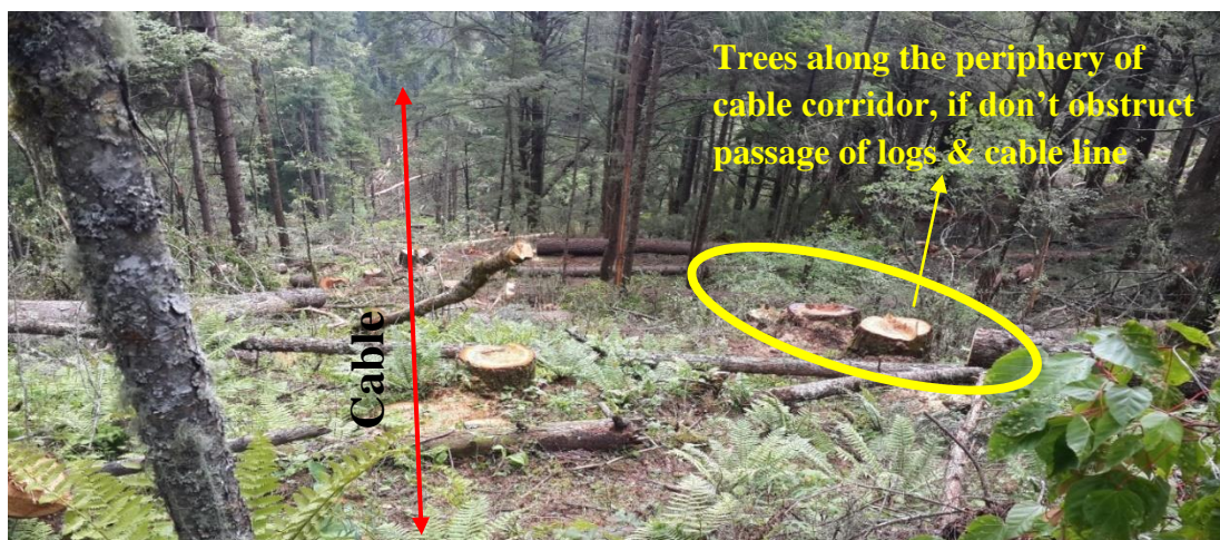
Figure 8: Cable corridor and felling of trees along the periphery
