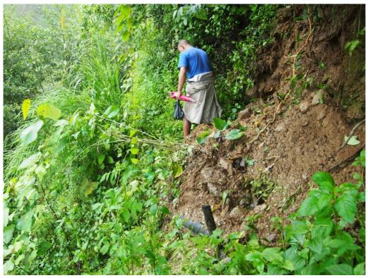
Figure 16: Landslips along irrigation channels
