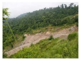
*Figure 7 : Massive landslide along the highway in Khagochen*
