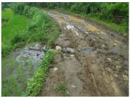
*Figure 18: farm road cut slope failure*
