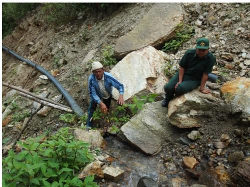
*Figure 14: Temporary irrigation channel intake in landslide along upper Balaychhu*
