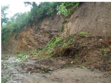
Figure 18: farm road cut slope failure
