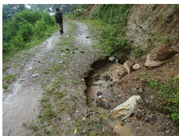
Figure 19: Improper water drainage
