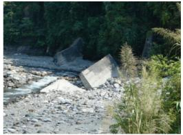
Figure 1:Groynes constructed (and subsequently destroyed by high river flows) in an unsuccessful attempt to train the river away from the BFAL factory site
