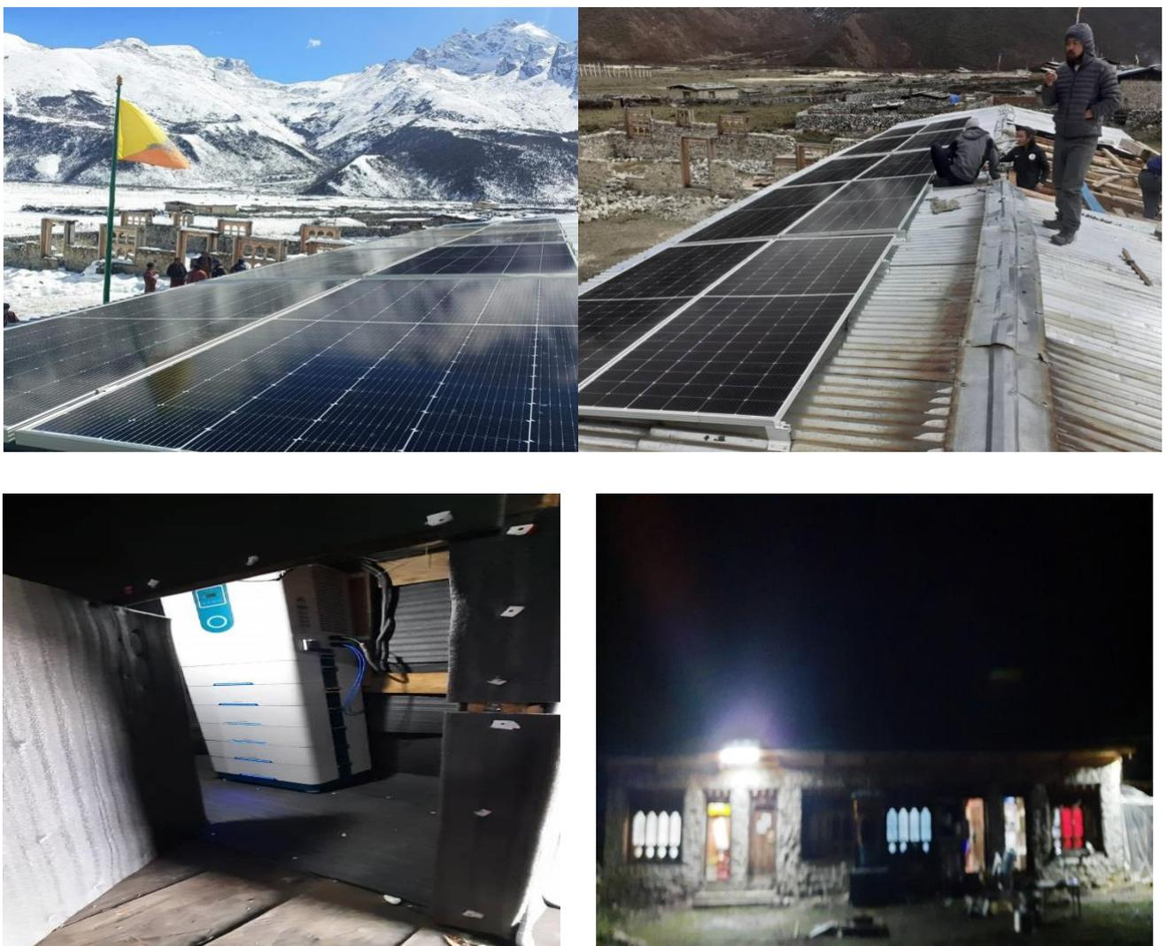
Figure 12: Solar PV plant at Lunana Extended Classroom (Yak in Classroom)
