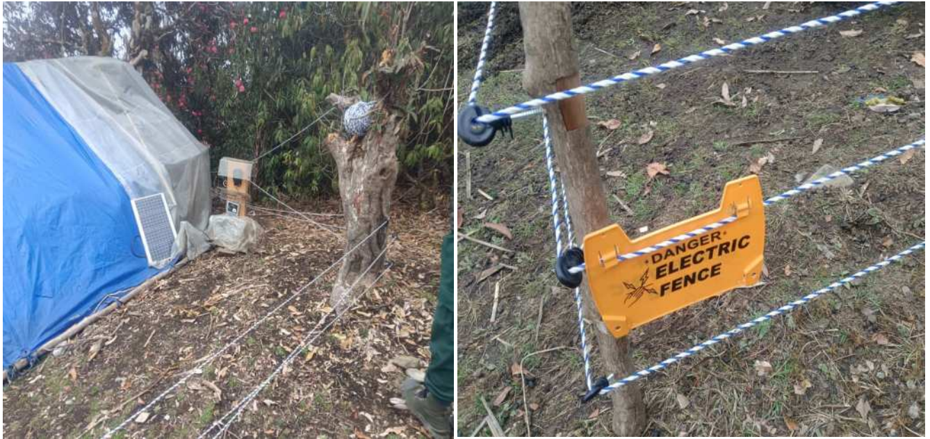
Figure 2. Corral fencing installed by NCD in Merak.
