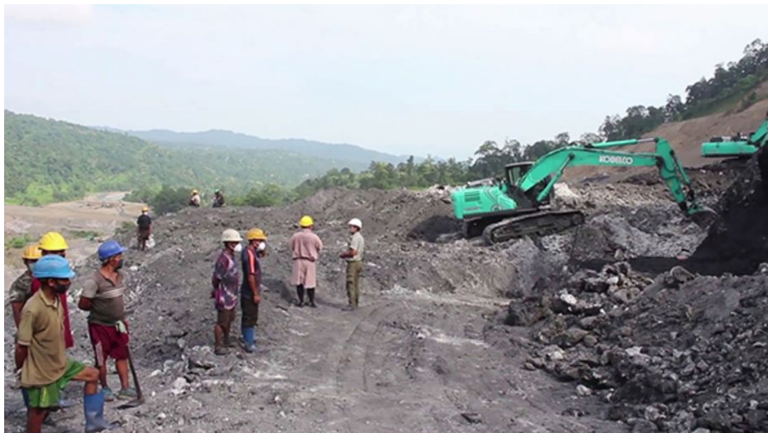
Figure 64: River-bed Materials dredging
